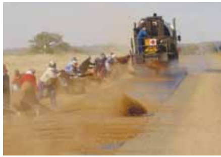
Spreading Natural Gravel by Hand in Otta Seal
