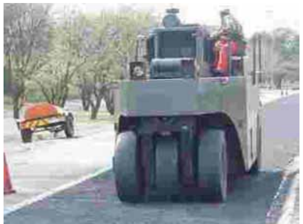
Compaction by a Pneumatic Roller
