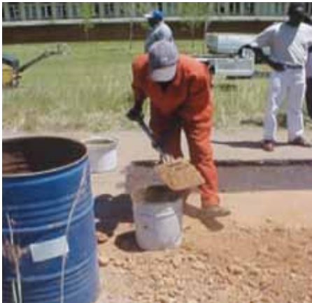
Batching aggregate, lime and cement
