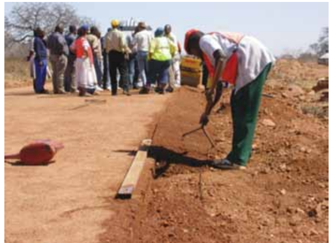
Edge Cladding of Based Layer
