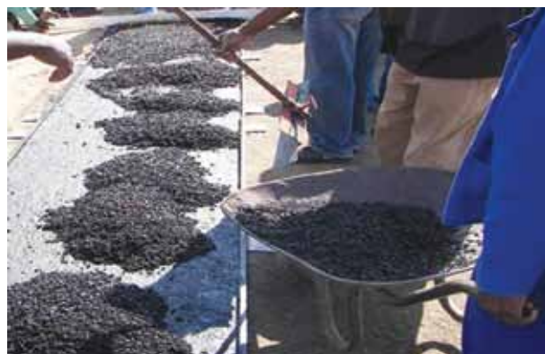
Spotting the asphalt
