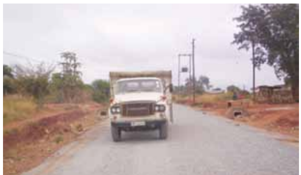
Loaded Tipper Trucks assisting in compaction
