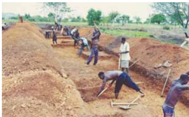
Excavation and stockpiling to create a loading bay
