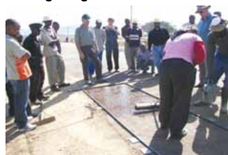
Application of tack coat
