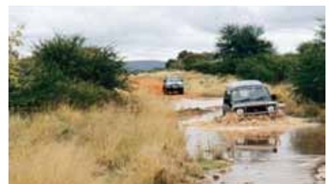
Roads without maintenance
