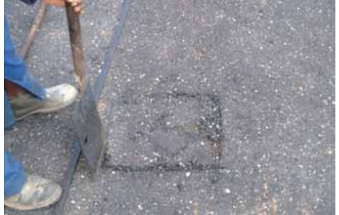
Trim the pothole area
