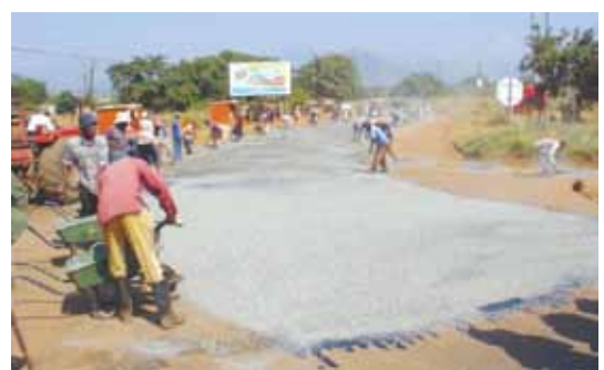
Slow spreading rate of aggregates by hand
