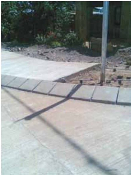
Completed UTRCP sections
