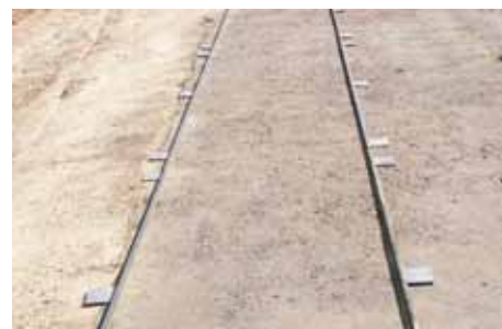
Placing the guard rails
