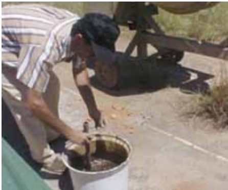
Mix remaining water and emulsion and add
