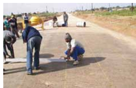
Marking position of guard rails
