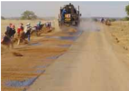
Spreading Natural Gravel by Hand in Otta Seal
