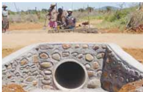
Stone pitched culvert wing wall
