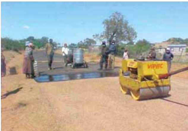
Compaction of Natural Sand Sealed Section
