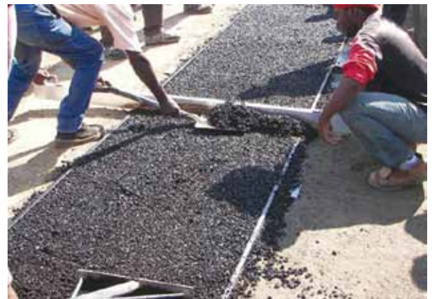
Screeding the asphalt
