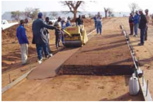
Compaction of ETB layer
