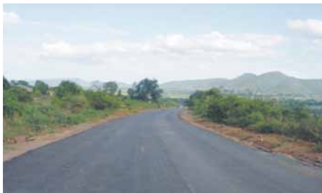
Completed asphalt sealed sections
