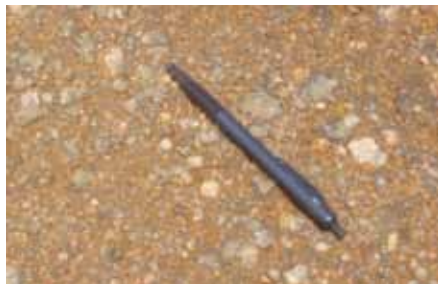
Compacted natural gravel Otta Seal
