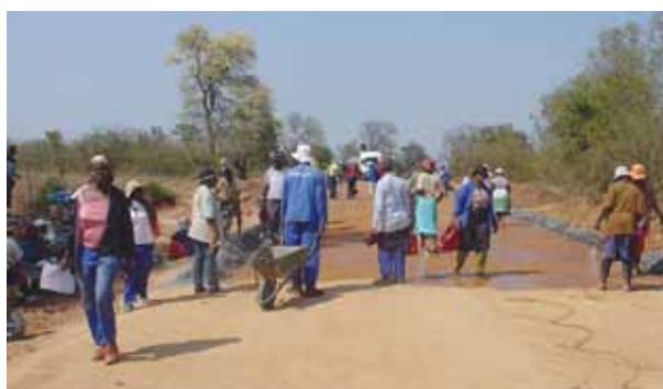
Watering the base Surface
