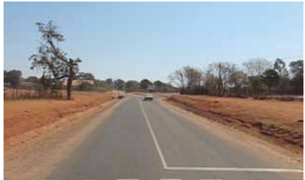
A completed Otta Seal section
