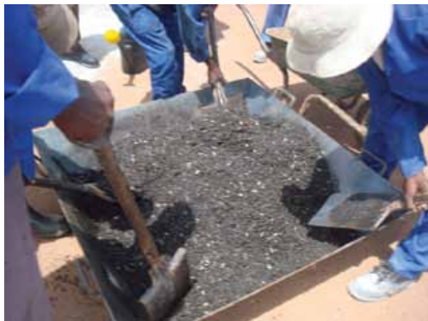
In-situ hand-mixing of asphalt
