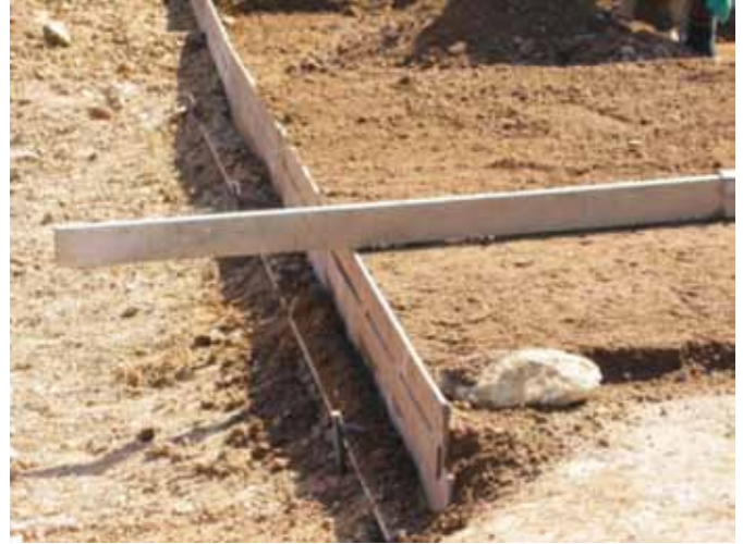
Use of screed board to level spread Base Layer
